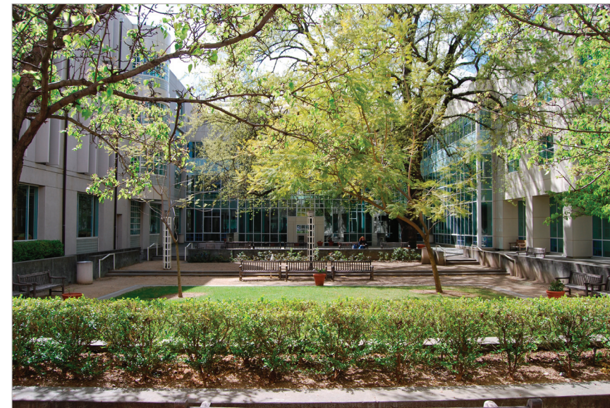
The west addition to Shields Library fully enclosed the original courtyard which includes a heritage oak tree that provides shading.
