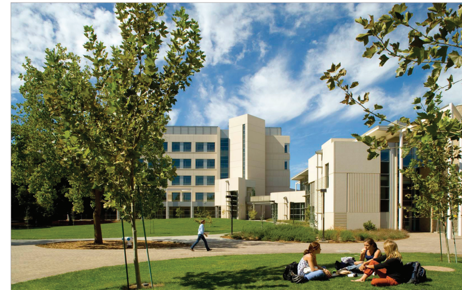
Health Sciences District, southern end of Tupper Corridor, in new open space framed by a research lab building, a teaching hospital, and a classroom building
