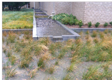
Functional expression of natural system: Valley Hall stormwater feature
