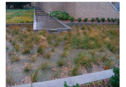
Local On-site Infiltration Basin: Small-scale site solutions offer the opportunity to educate as well as manage runoff of small sites. The size of the Davis campus makes larger overland surface solutions possible as well.
