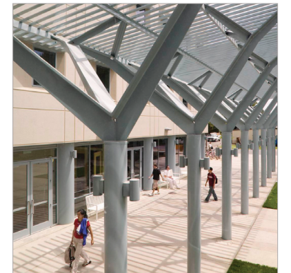
The openness and height of this trellis together make it unable to offer adequate shelter from the strong Central Valley sun.
