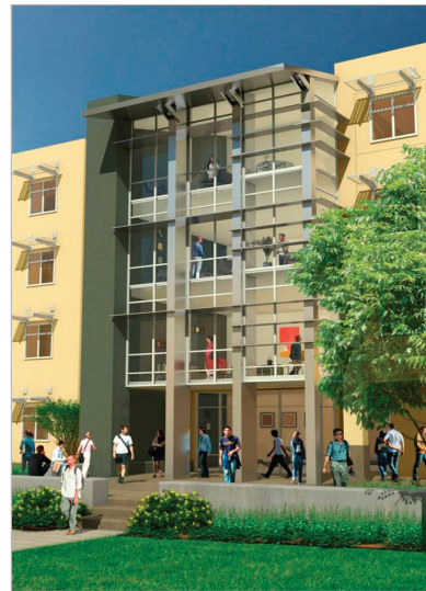
The seat walls at this entry provide a welcoming place to meet or wait
