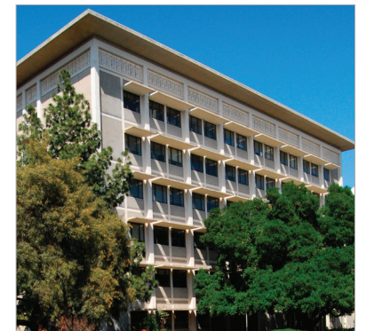
Sun control on windows (Storer Hall)
