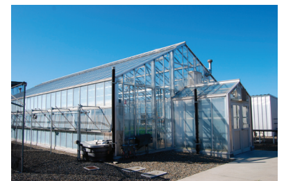
An example of the range of colors and materials for the agricultural vernacular buildings on the south and west campus.
